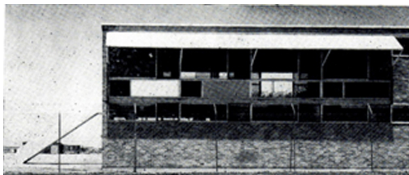
Fig. 1. Permanent Awning Projection on North Facade of Amenities Building, Banksmeadow, Sydney. Made of Zinc Anneal Steel.
